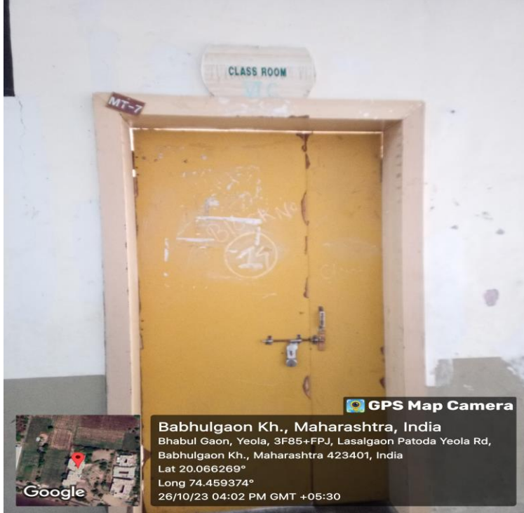
Classrooms (TF)- Classroom MT-7-
